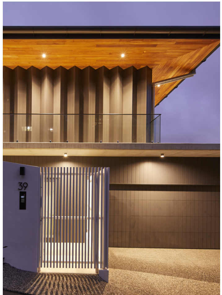
VANQUISH JOE ADSETT ARCHITECTS WITH SOLAIRE PROPERTIES AND ECO LATERAL ENVIRONMENTAL CONSULTANTS
